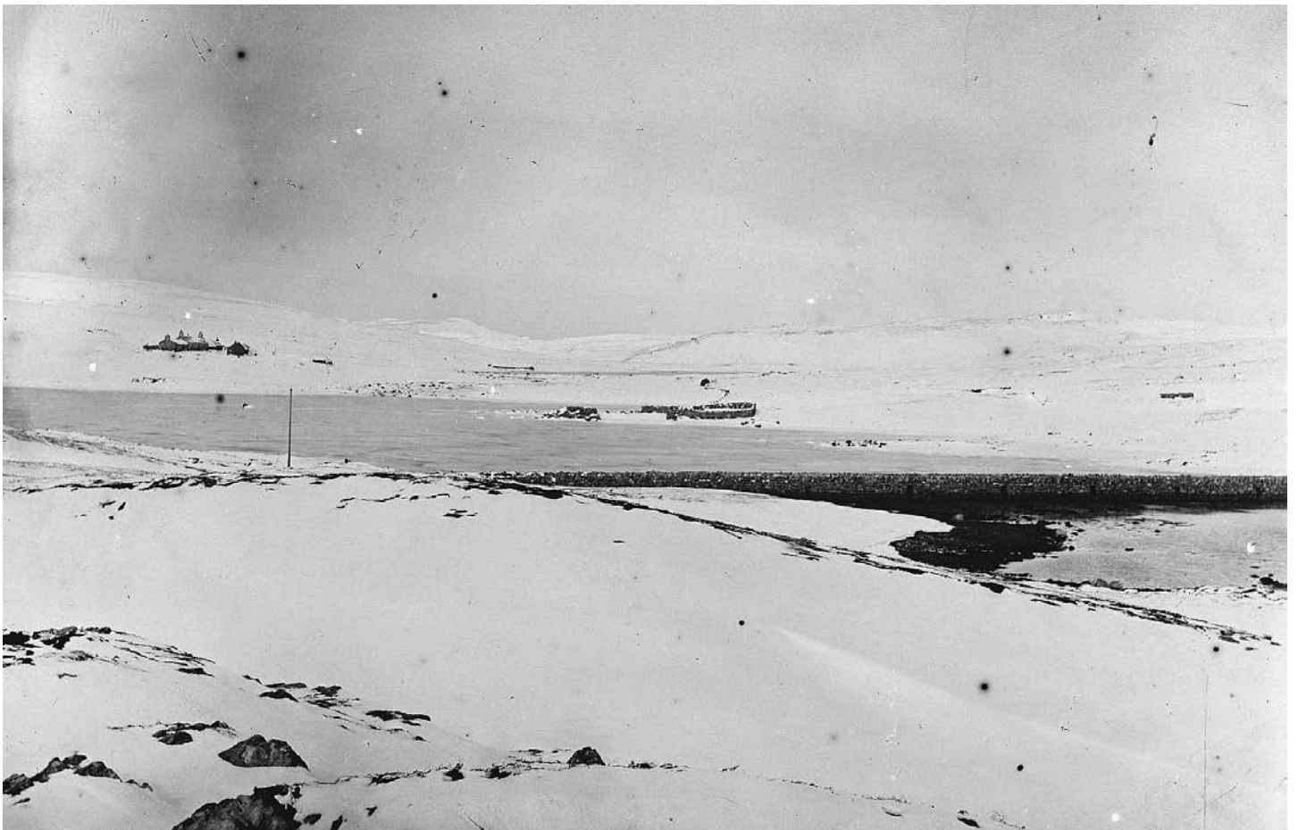
The Royal Engineers built the bridge at the head of the Voe of Bruland around 1850. Here it is fifty years later, with Brouster in the distance.
