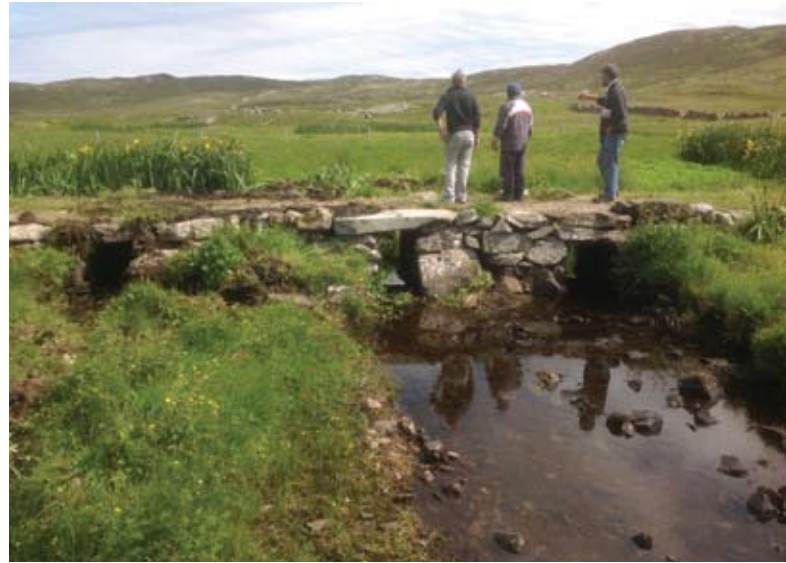
Bridge on the track near Brouster, Waas, restored in 2014.
