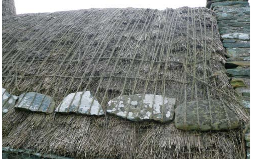
Coir rope used to hold down thatch; vertical strands hold the weights, while horizontal ones hold the latter in position.
