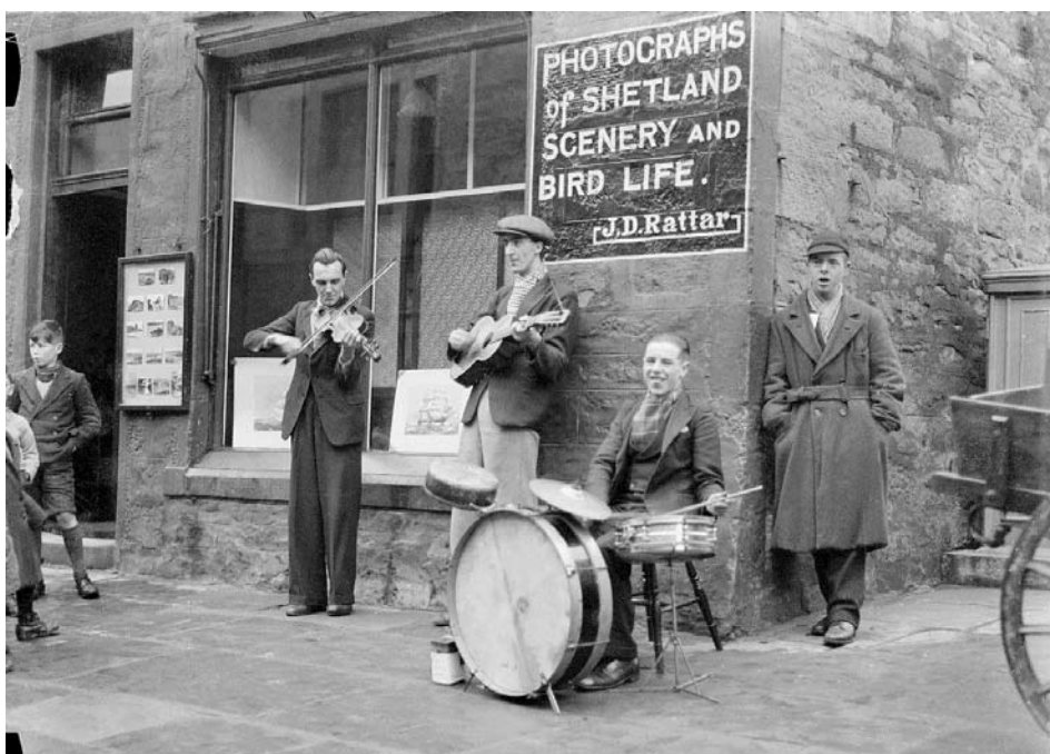
This photographer once traded in signwriting, so was able to paint his sign on the masonry of 175 Commercial Street himself.
