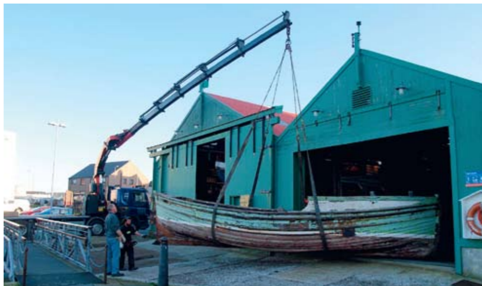
The Oceanic 's lifeboat is 29 feet long, and some nimble crane work was needed to get her into the boatshed.
